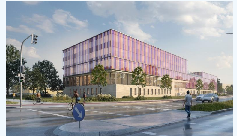
William B. Kannel Center for Community Medicine (under construction)
